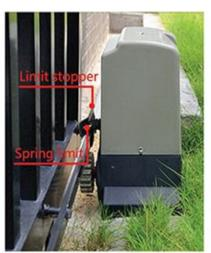
Move the gate manually to the open limit and close limit, mark the points on the rack, then, fix the limit stoppers or magnets at the limit points on the rack
